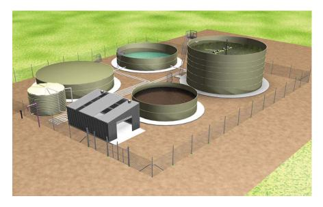
reactor basin, after settling the decanter removes the clear water from just below the top of the water column by gravity using a solids excluding floating decanter to the Decant Tank.
