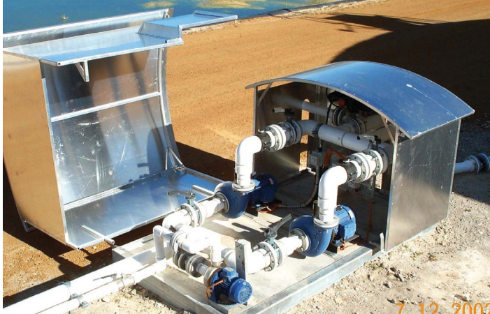
All automatic control valves and transfer pumps were pre manufactured and mounted on a skid providing a compact unit and easy installation.
